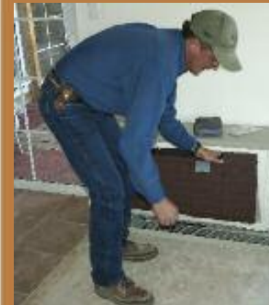
A co-op member services employee makes adjustments to a consumer's ETS unit.
