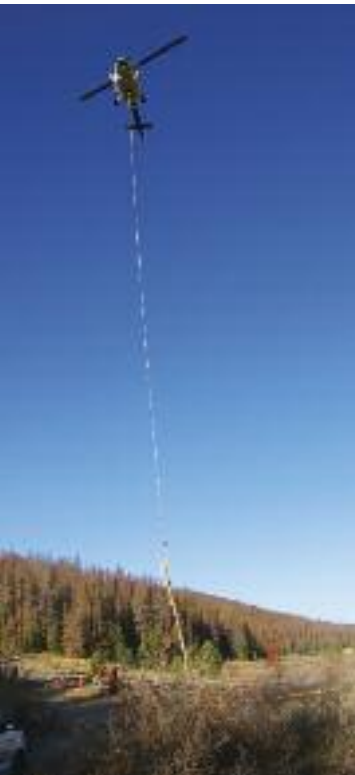
Contract heli-logging doesn’t come cheap, but is necessary in some of the less accessible right-of-way wilderness areas like this one shown in Mountain Parks Electric’s service territory. Photo by Les Shankland.
